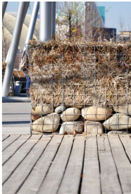
Gabion walls with biogenic materials
