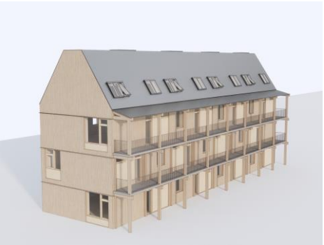
Balcony acces - high-strength concrete
